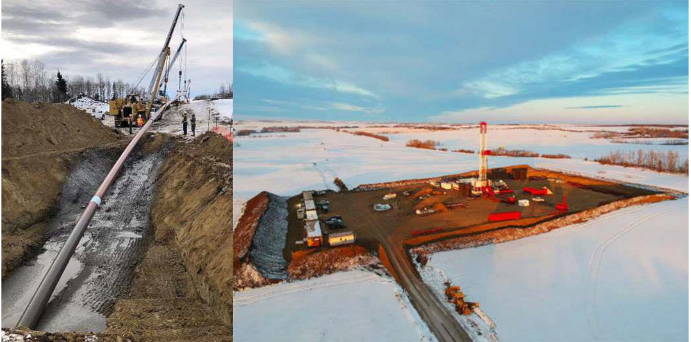
ACTL Pipelining and Injection Well Drilling at Clive
