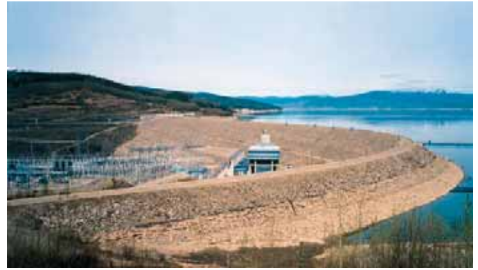
Hydroelectric Power Grid, W.A.C. Bennett Dam (AENV)
