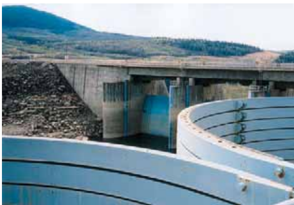
W.A.C. Bennett Dam (AENV)
