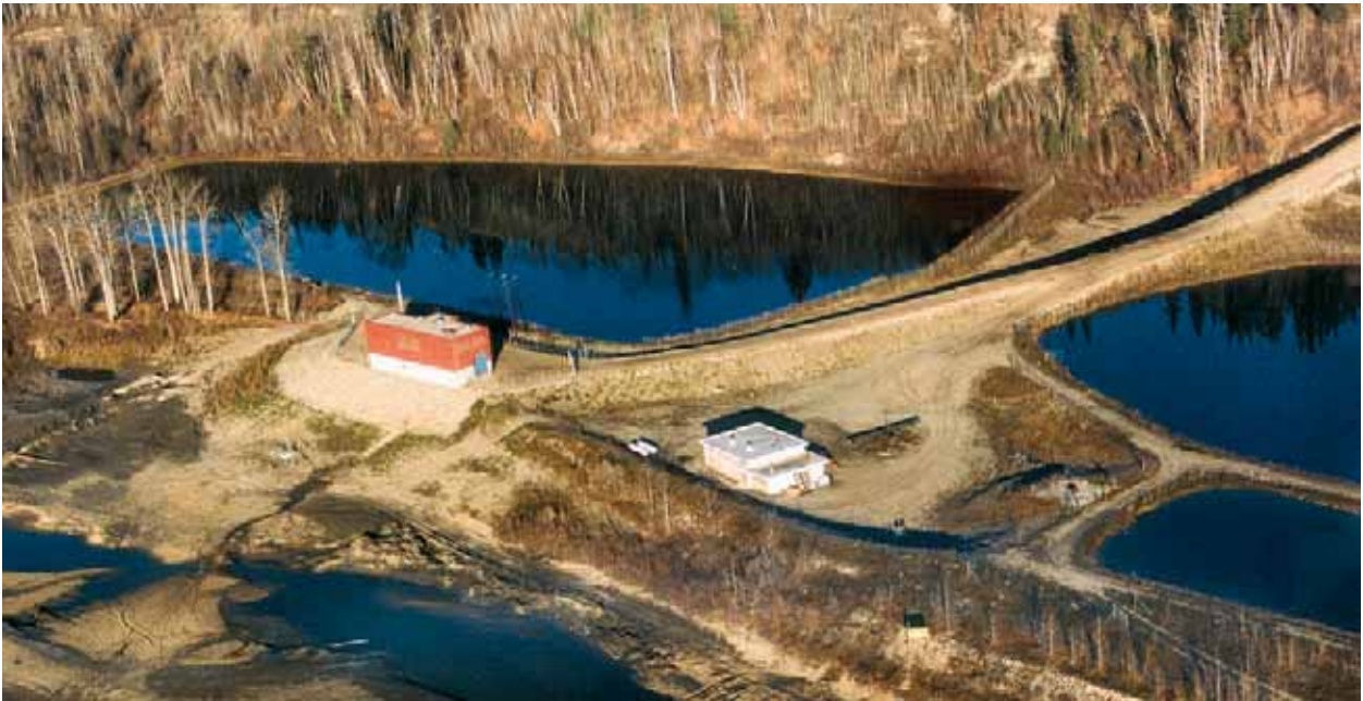
Grande Prairie's Old Water Treatment Plant and New Raw Water Pumphouse on Wapiti River (AENV)
