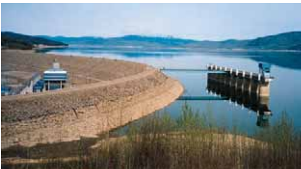
Williston Reservoir, W.A.C. Bennett Dam (AENV)
