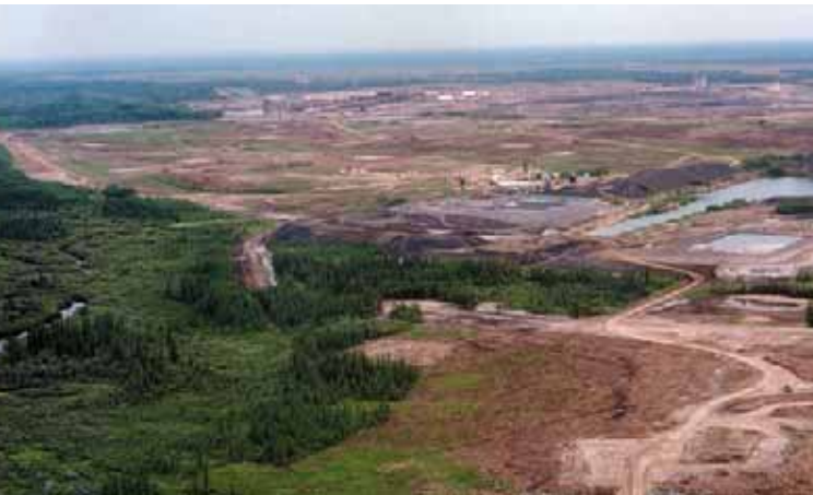
Albian Oil Sands Construction Site (AENV)
