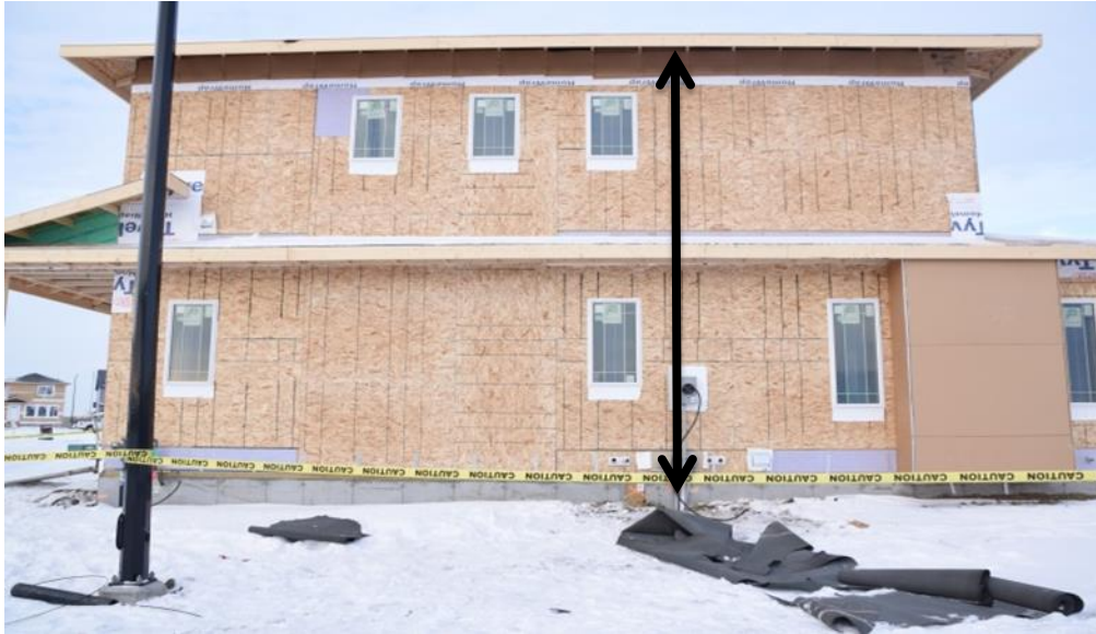
Figure 2- The roof height approx. 6.7 metres.
