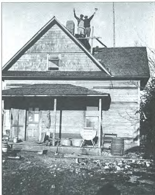
Chimney under construction at the O'Bryant/Metcalf Residence in 1932. (Price Family)
