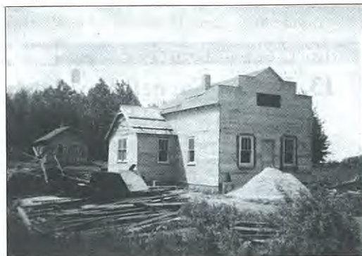
The North Hill Store under construction in c. 1943. (RDDA)
