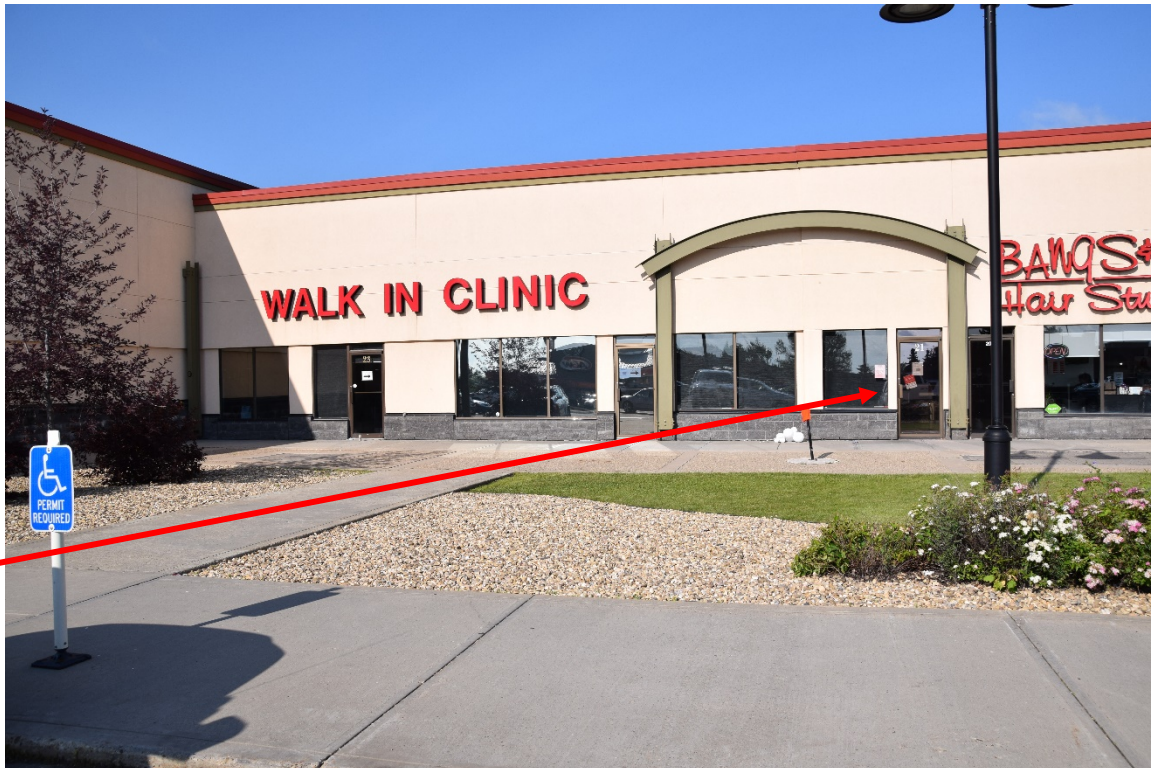
Figure 1. Entrance to Village Mall Medical Clinic A. Public entryway
