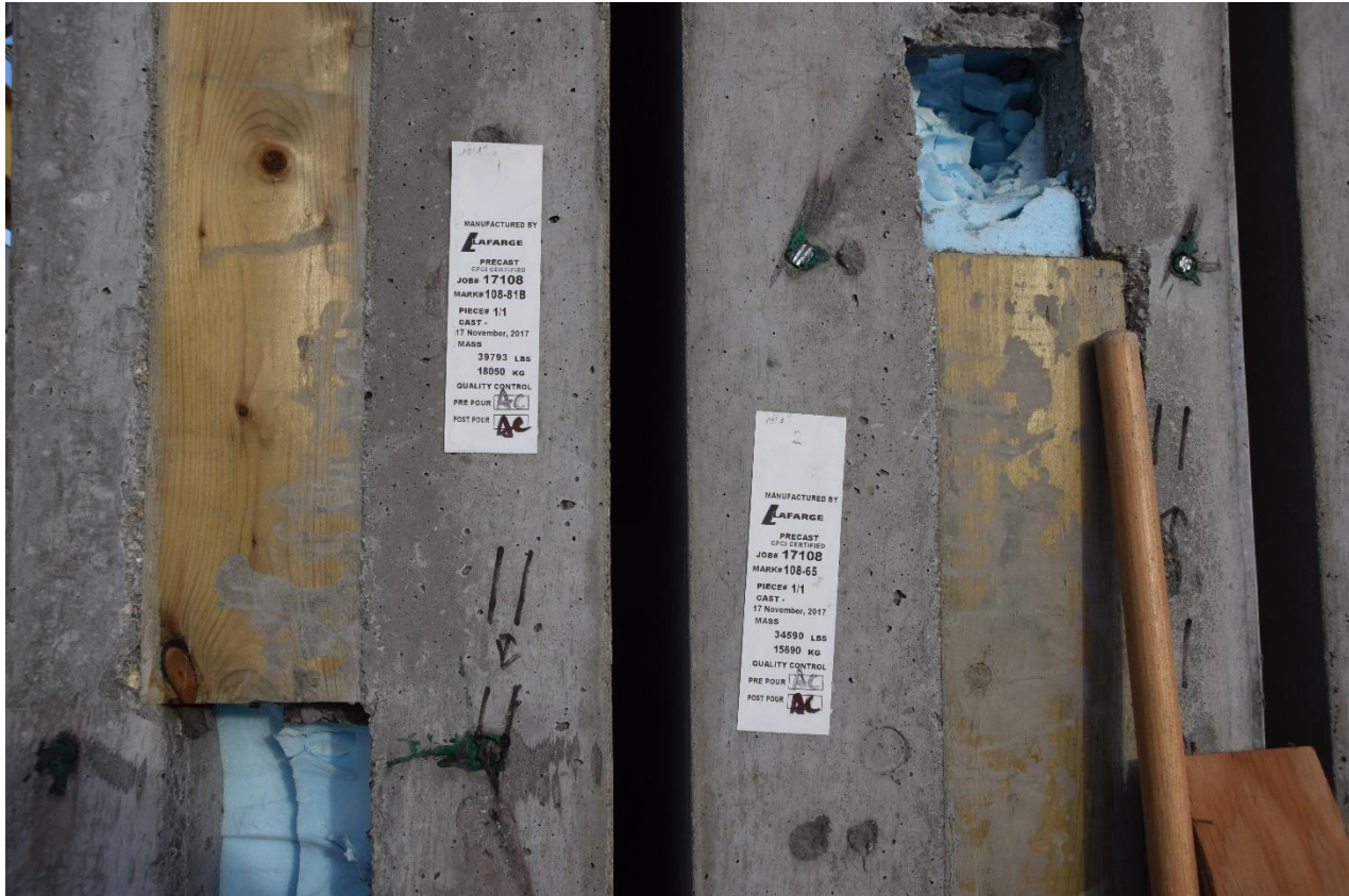
Figure 3. Manufacturing labels affixed to Insulcore panels stored in the gantry crane bay
