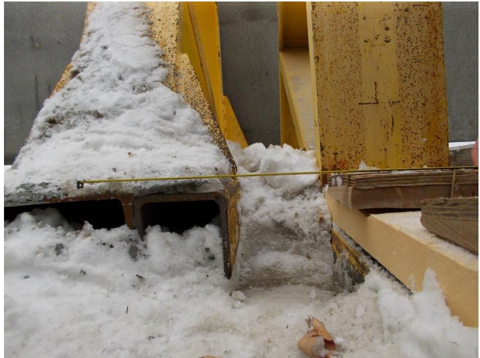
Figure 14. Ice and snow on foot of east facing storage frame on north end of aisle involved in the incident
