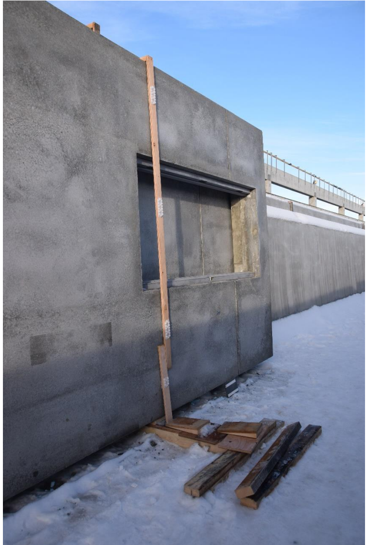
Figure 9. Dunnage used to level and separate precast panels
