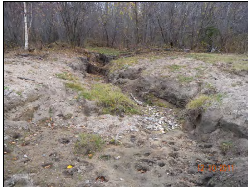
Dry channel of SG9-1, October 12, 2011
