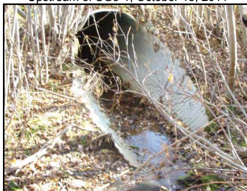
Upstream end of SG5-1 culvert at highway, October 15, 2011
