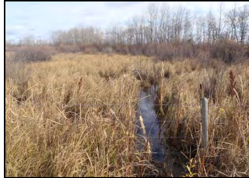
Upstream of culvert at SM3a-1, October 14, 2012
