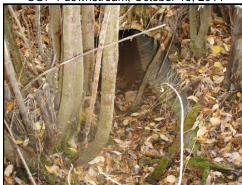
SG7-1 culvert, October 15, 2011
