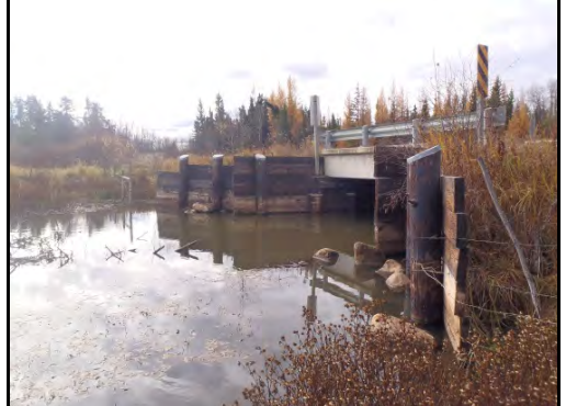
Culvert at MOC-2, October 14, 2011
