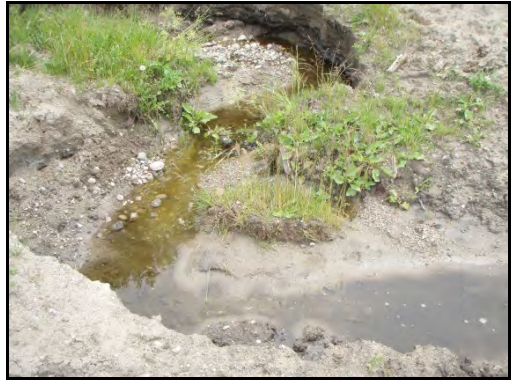
Stagnant water at outlet of SG8-1, July 12, 2011
