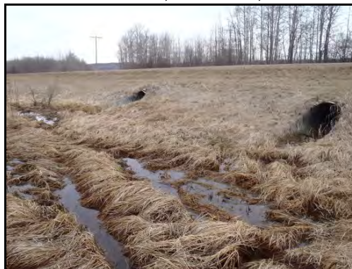
New channels through grass to small culverts, May 5, 2012
