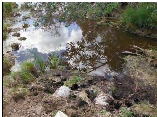
Culvert under cutline, SG21-1, August 8, 2013
