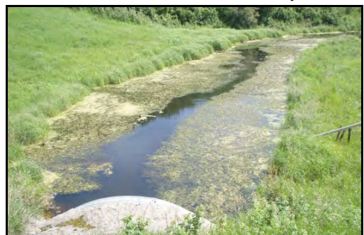
Upstream end GAC-1 culvert, July 14, 2011
