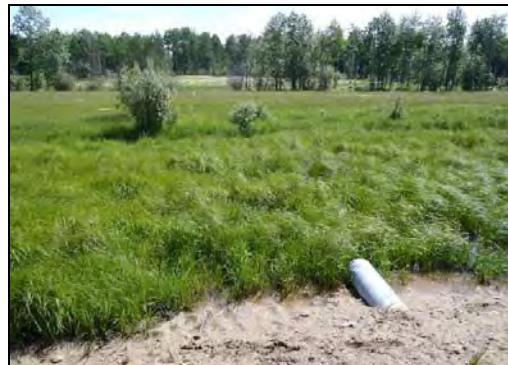
Culvert at SG4-4, June 19, 2013
