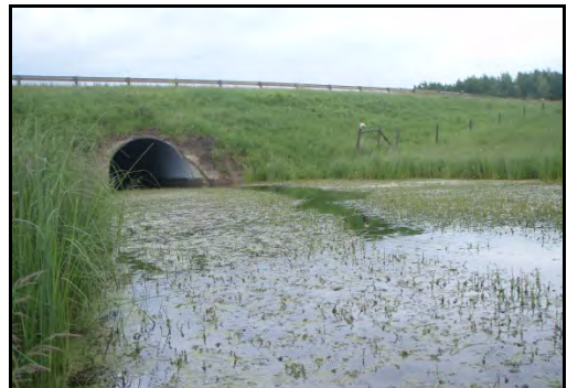
Downstream end of GAC-1 culvert, July 14, 2011
