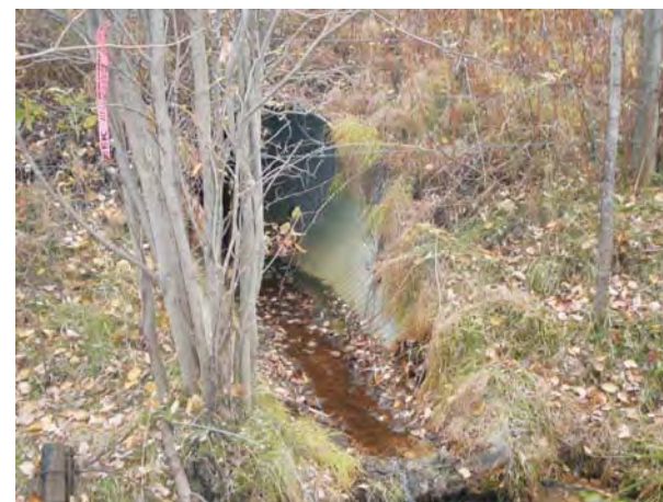
Culvert upstream of cross section
