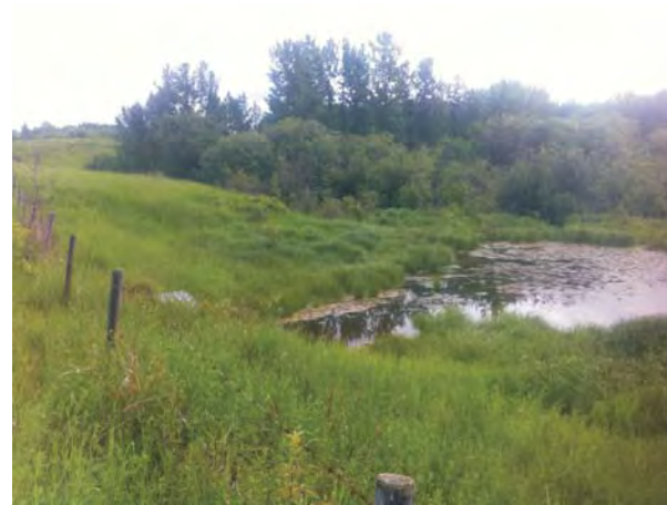
Culvert upstream of cross section
