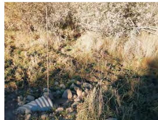
View of culvert inlet
