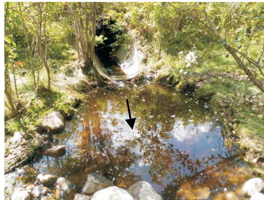
View of culvert at site
