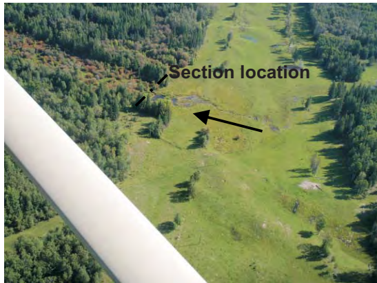
Aerial view of site
