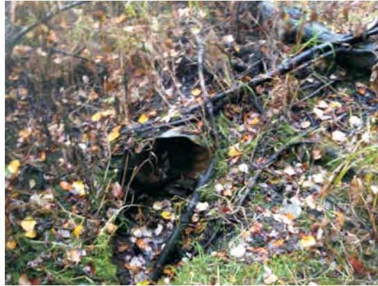
View of culvert at site
