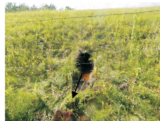
View of culvert looking upstream
