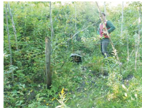
Culvert upstream of road
