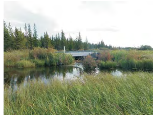
View of cross section upstream of bridge
