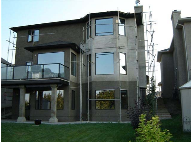
Repair to a wall facade
