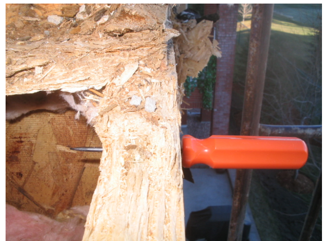
Screw driver through support member
