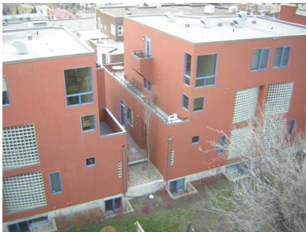
Exterior façade before removal
