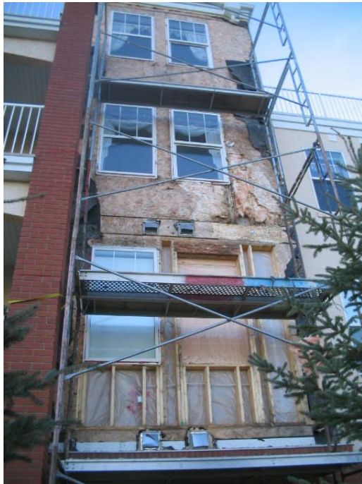
Repair to affected wall
