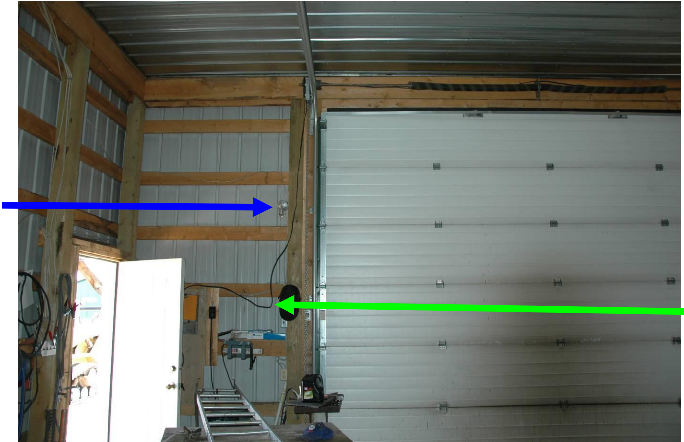
Photograph 4 – Re-creation of the scene by the employer (*****)) shows the approximate location of the ladder lying on top of a wooden work bench, in relation to the wire the Foreman (*****)) was planning to secure. The green arrow points to the bend in the electrical wire. The blue arrow points to the light fixture with a broken bulb.
