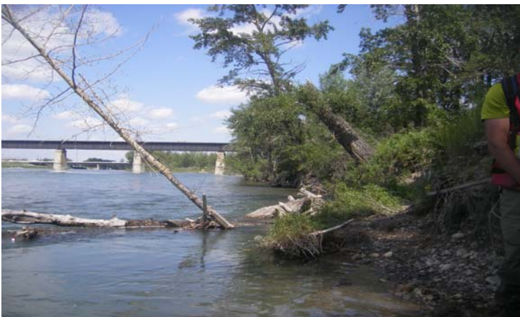
3L looking upstream
