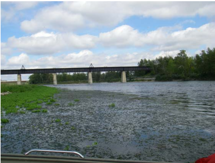
3R looking upstream
