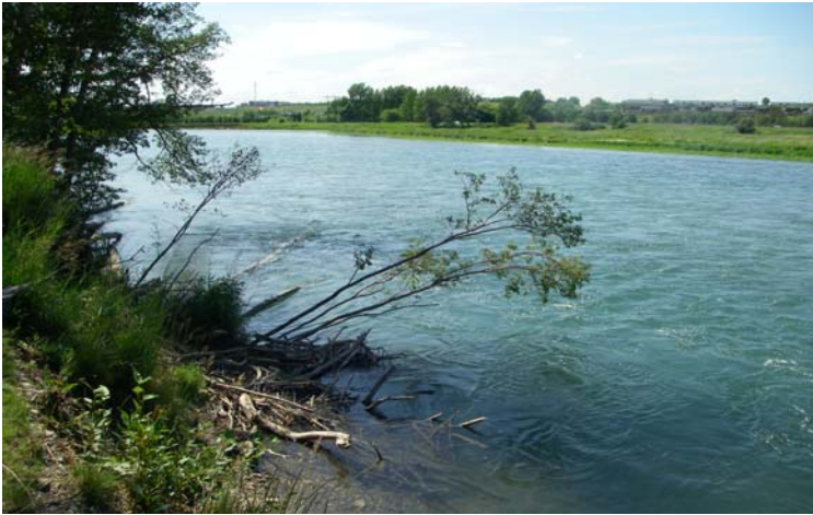
3L looking downstream
