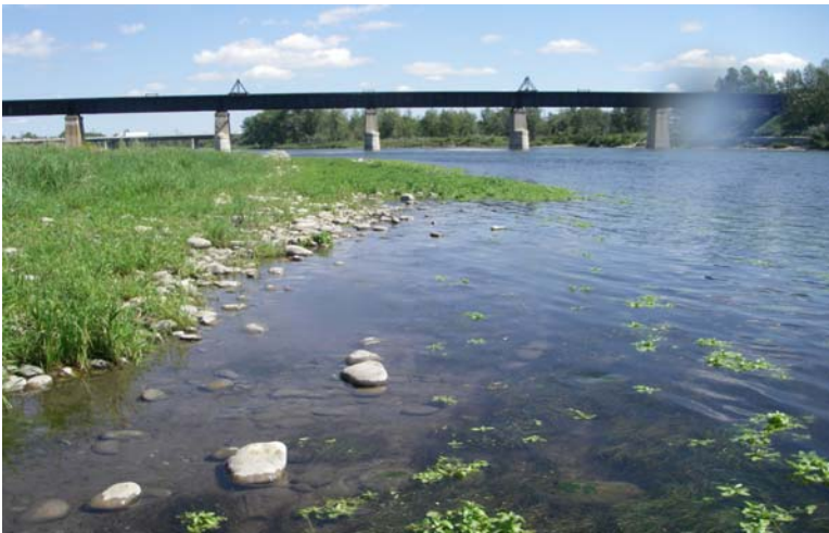
3R looking upstream
