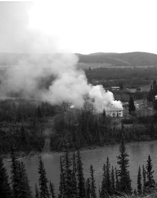
The Ghost Dam exercise seen from a distance
