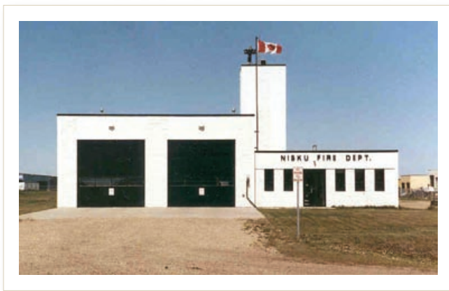
Nisku Industrial Park's new fire station – 1976
