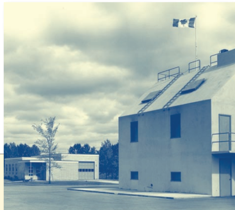
The original structures at the Alberta Fire Training School.
