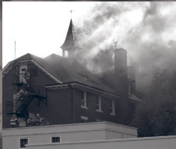
June 18, 2003 fire at Michener Service building in Red Deer
