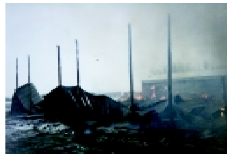
Wooden supporting poles and metal sheets, which were the walls, remain after a fire destroyed a flax-bale storage building and adjacent buildings.
