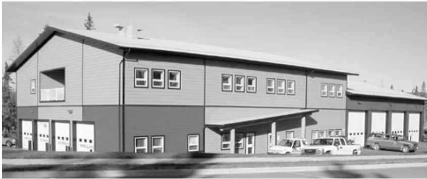
The Hinton Fire Department's new home, which also houses the town's ambulance service
