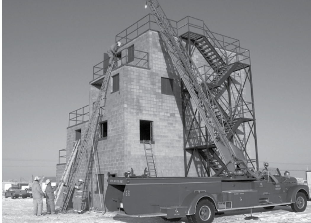
Trainees go through the paces at the Brooks Regional Fire Training Facility
