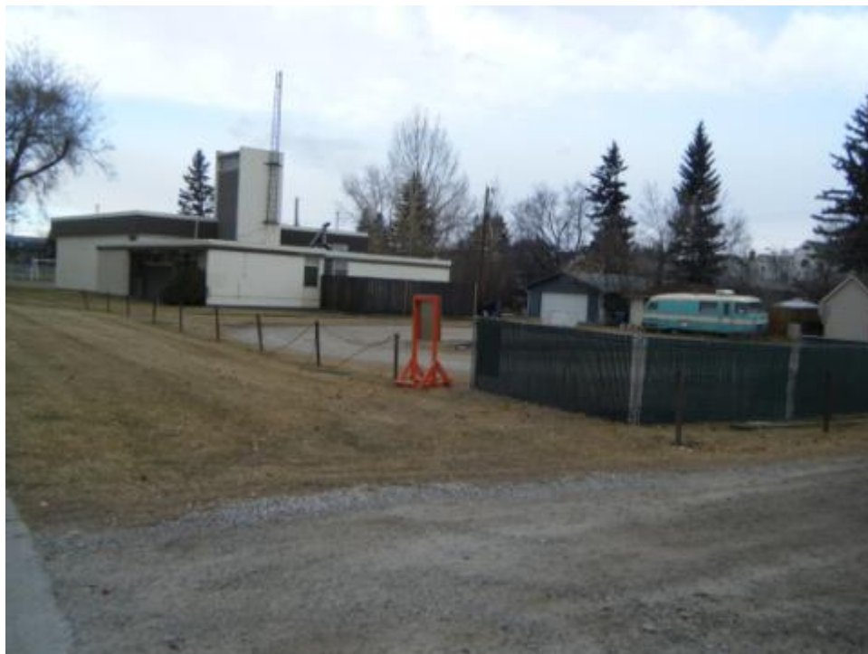
↑ Photograph 6 EMS Firehall looking northwest.
