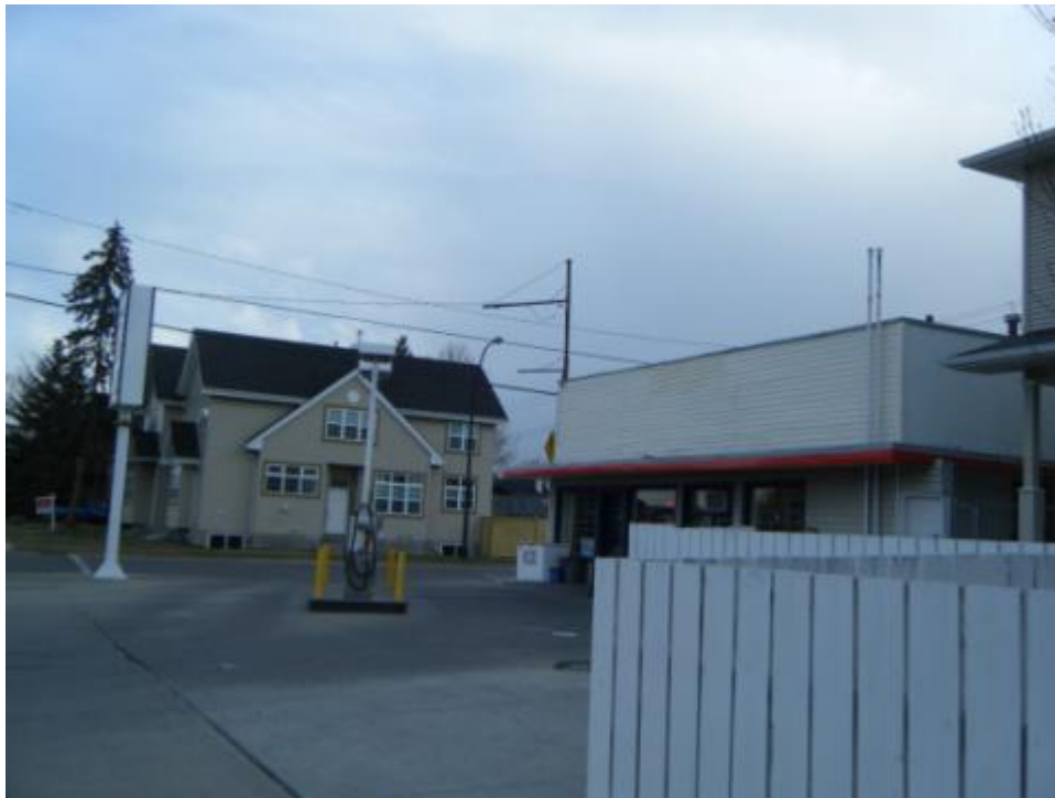
↑ Photograph 11 Gas pumps at Westmount Auto Centre, looking east.
