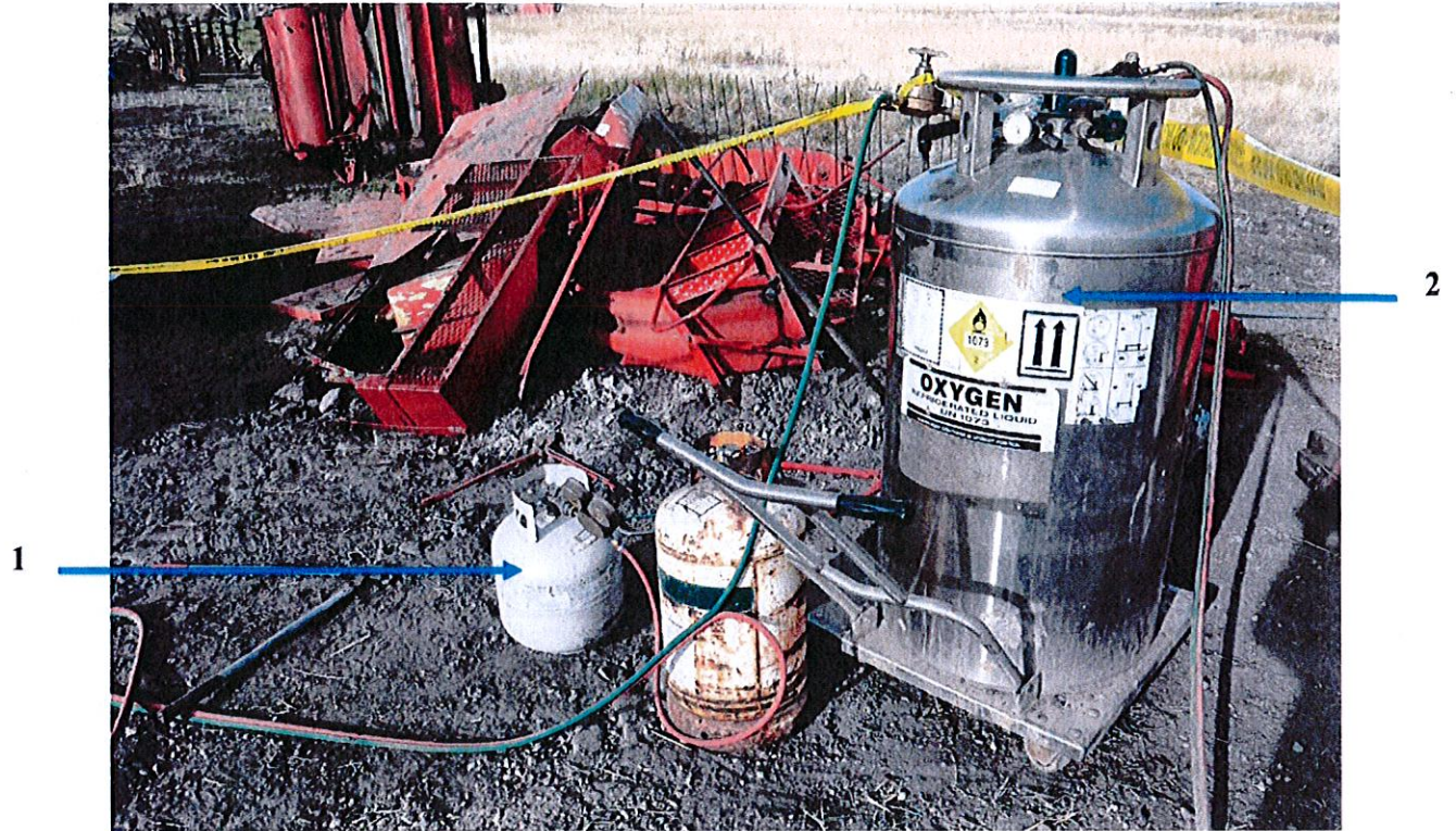
Photograph #5: Shows the gas cylinders used for torch cutting.
