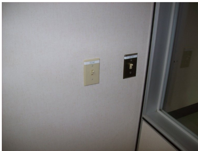
Typical line voltage toggle switches.
