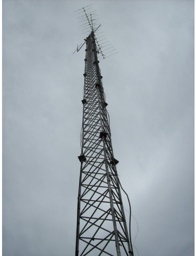
Radio antenna located adjacent to the Health Care Building
