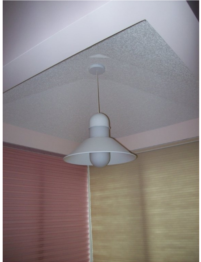
Typical incandescent pendant fixture
