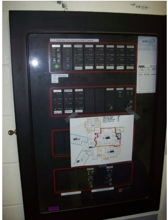
Simplex FACP dating from 1976 Const.
