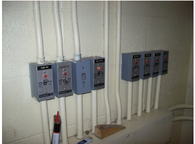
Typical Westinghouse manual motor starters
