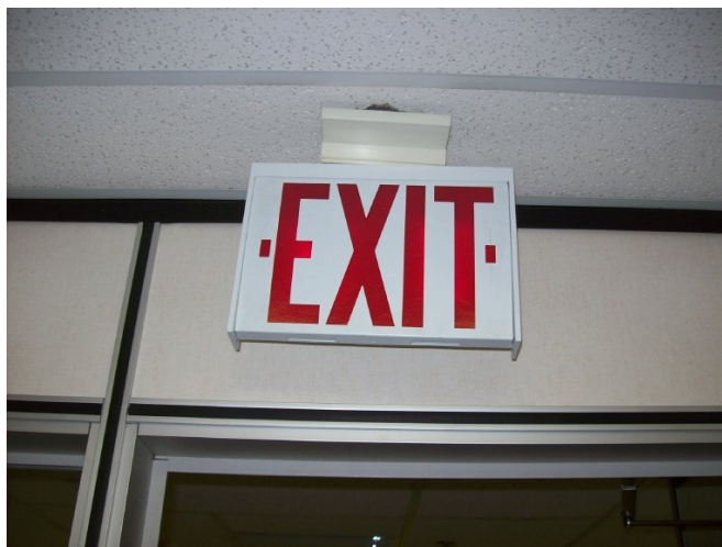
Typical 1975 exit signs.
