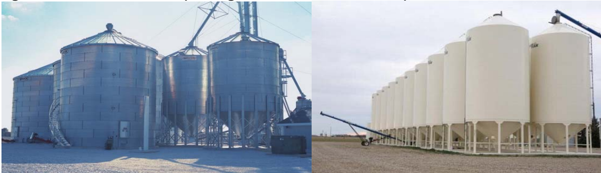
Figure 5. Steel Grain Bins (Corrugated and Smooth Walled)
