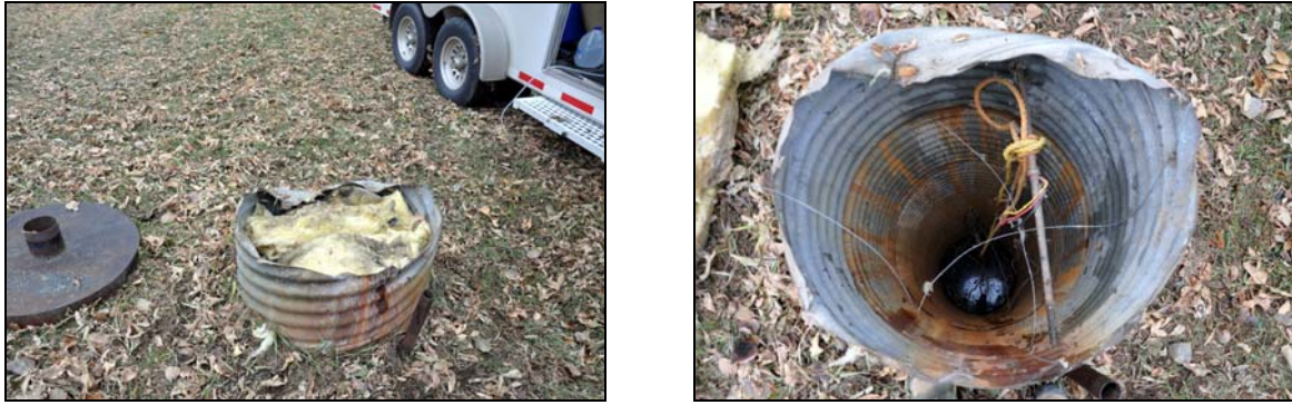
Figure 12: Well 5 located on Site 1.
