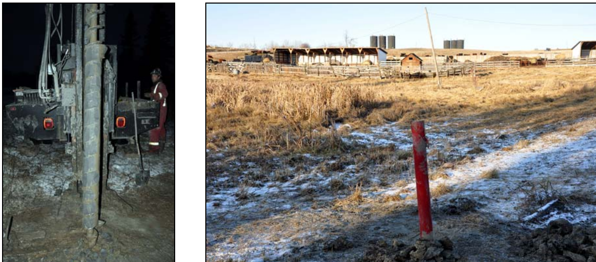
Figure 22: Image to the left shows the drilling of MW1 on Site 2. Image to the right shows MW1 with the feed lot and energy well batteries in the background. Well 1 is located 8 m directly to the east of MW1.
