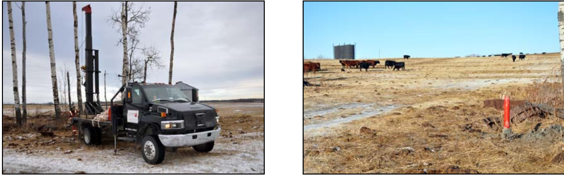
Figure 23: Image to the left shows the installation of MW2 on Site 2. Image to the right shows the completed well. Note the energy well battery in the background. Also to the north where the cattle are grazing is the fertilizer applied field.
