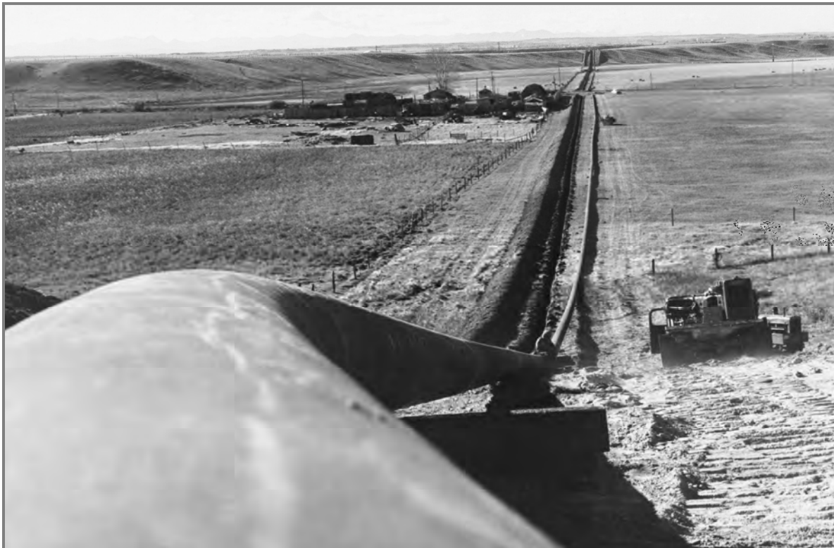
Laying of Gas Pipeline between Carbon and Calgary, Alberta. 1958
