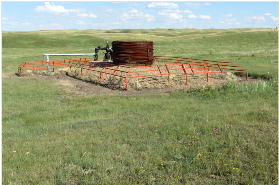
Minimal Disturbance Wellsite—Hand Hills
