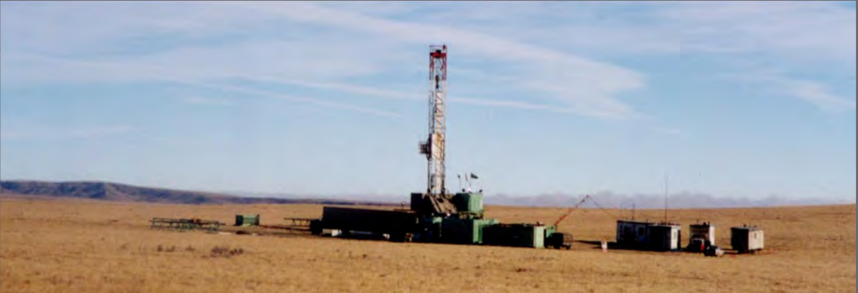
Reduced Disturbance Wellsite Construction During Dry Ground Conditions.
