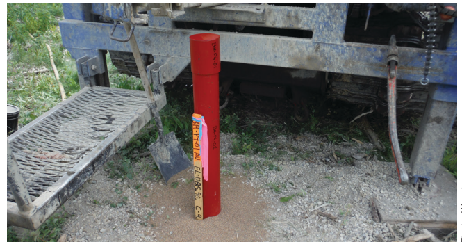
Example Standpipe installation with protective steel casing riser.
