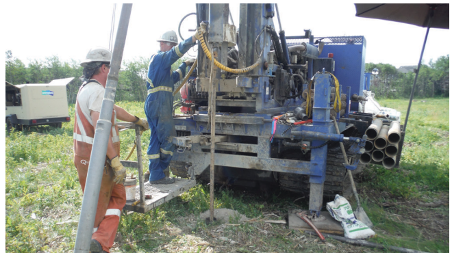
Example track-mounted downhole hammer drill with auxiliary air compressor (back left).
