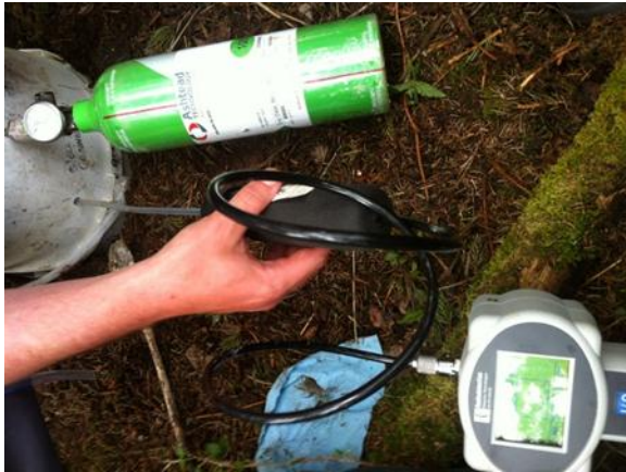
Figure 3.6-4: Leak Test (left photo) – Flushmount Vault (right photo)
