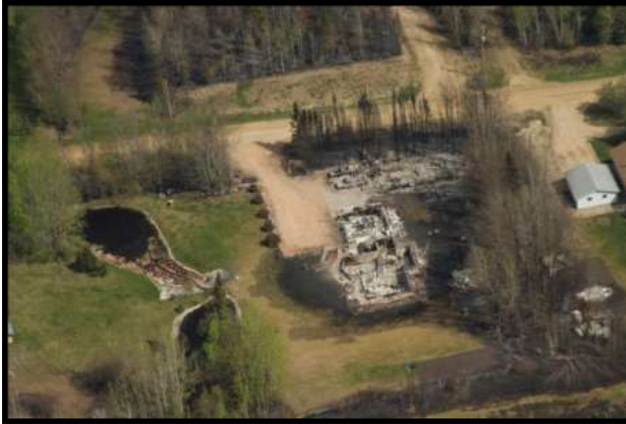
Figure 87 – Wildfire followed fuel accumulations along tree lines and ignited structures (Canyon Creek).
