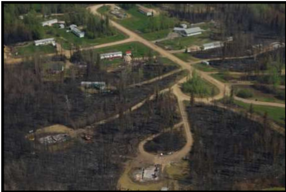
Figure 86 – Structures in close proximity to mixedwood (M1) fuels ignited by flame contact (Widewater).
