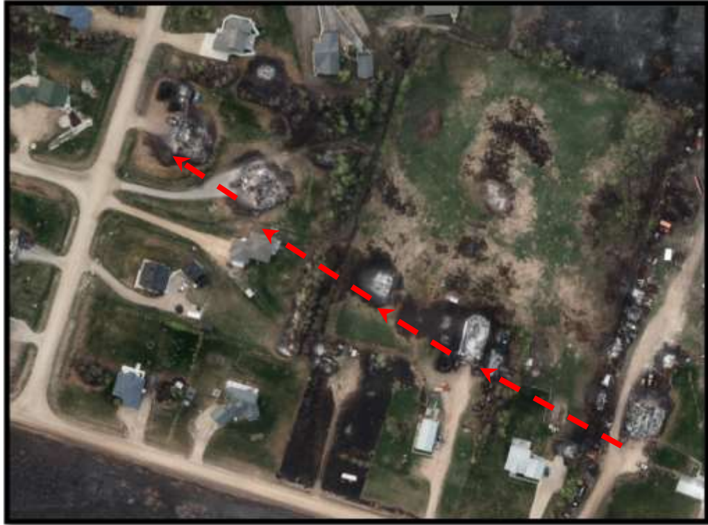
Figure 134 – Structure-to-structure firebrand transport ignited homes in conjunction with surface fire spread.
