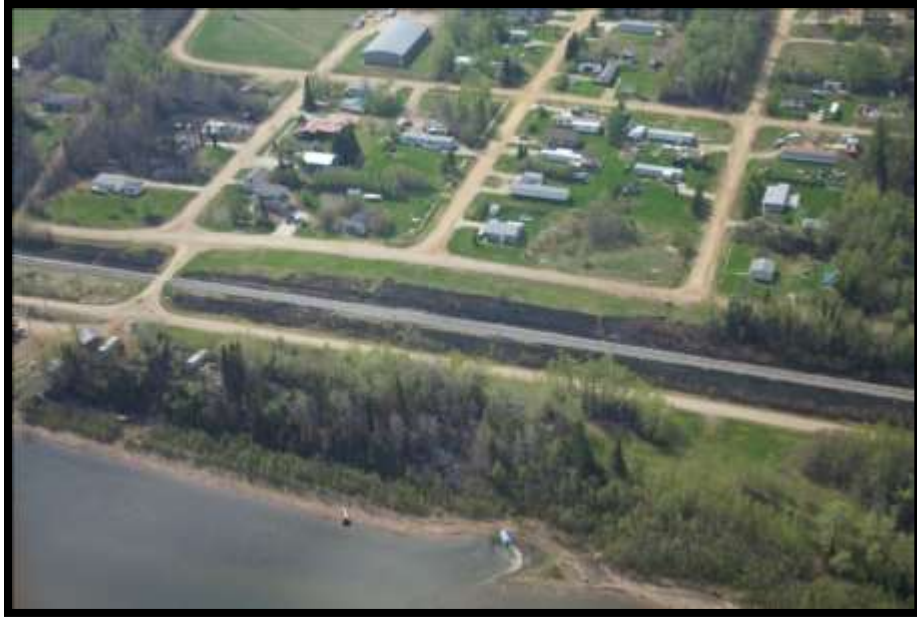
Figure 85 – Open areas of grass where fuel loading was reduced did not sustain wildfire spread. Evidence of wicking in grass accumulation along right-of-way (Canyon Creek) was noted.
