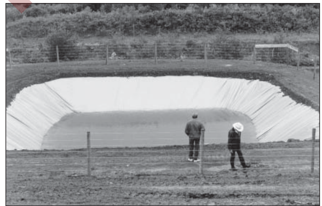
Figure 2. Elevated earthen reservoir with woven polyethylene liner
