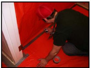
Worker Constructing Polyethylene Containment
