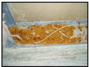
Water-Damaged (Rusted) Metal Bottom Plate
