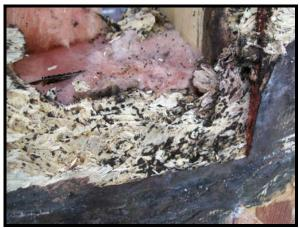
Mould-Contaminated Oriented Strand Board
