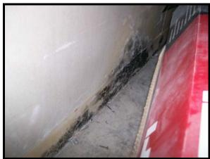
Mould Contaminated Drywall Behind Cardboard Box
