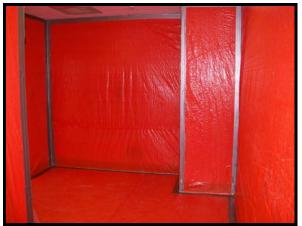
View of Polyethylene Containment using Orange Re-enforced Polyethylene
