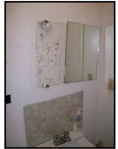
Mould-Contaminated Drywall Behind Mirror
