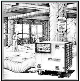
View of HEPA Negative Air Unit Inside a Containment
