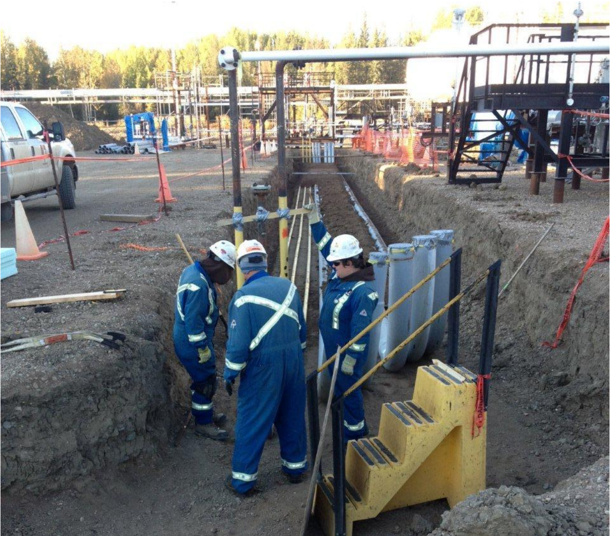
Figure 16: Underground Pipe Installation
