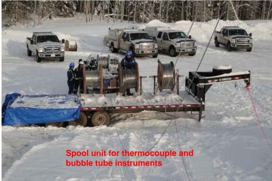
Figure 6: Well Site Photo during HW Completions Work (Cont'd)
