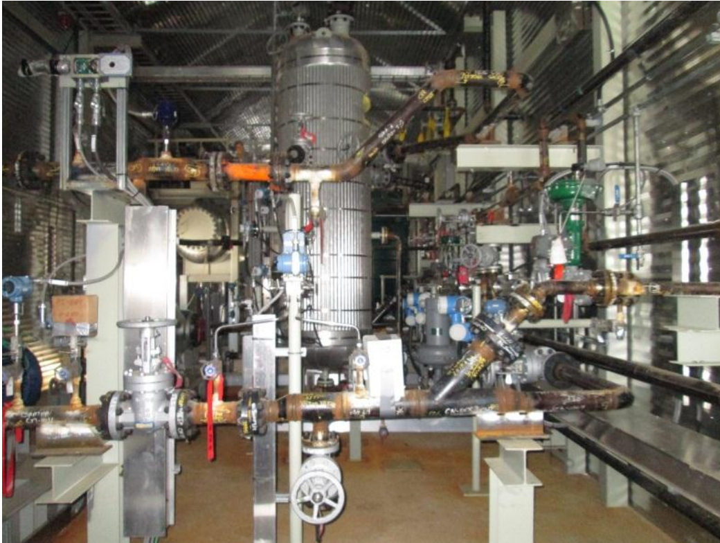
Figure 9: Interior of Production Building
