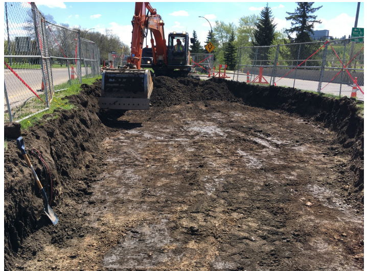
Figure 9. Removal of historic/contemporary overburden at FjPj-116.
