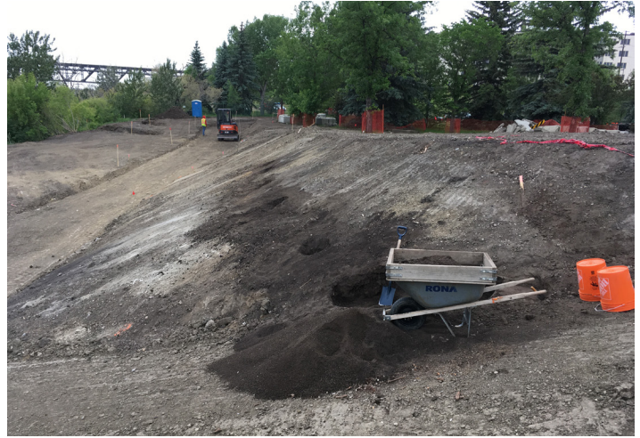
Figure 20. Shovel testing program west of access stairs.
