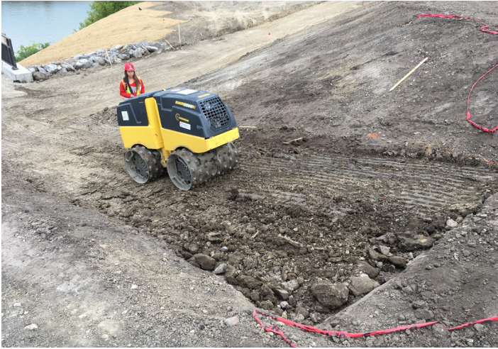
Figure 19. Packed clay foundation fill at access stairs.
