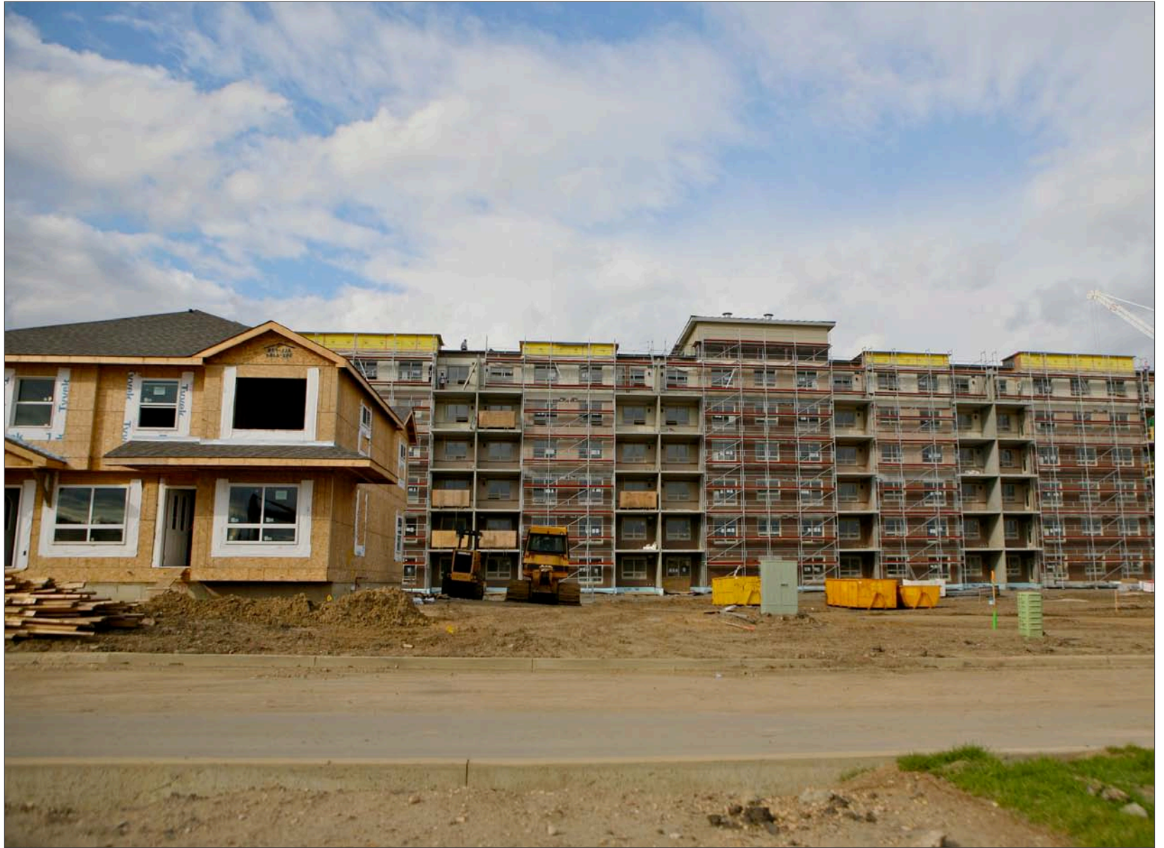
Construction of Low and Medium Density Housing in Fort McMurray
