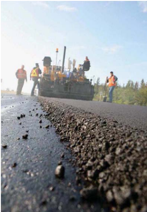
Figure 3: Highway Upgrading Near Fort McMurray
