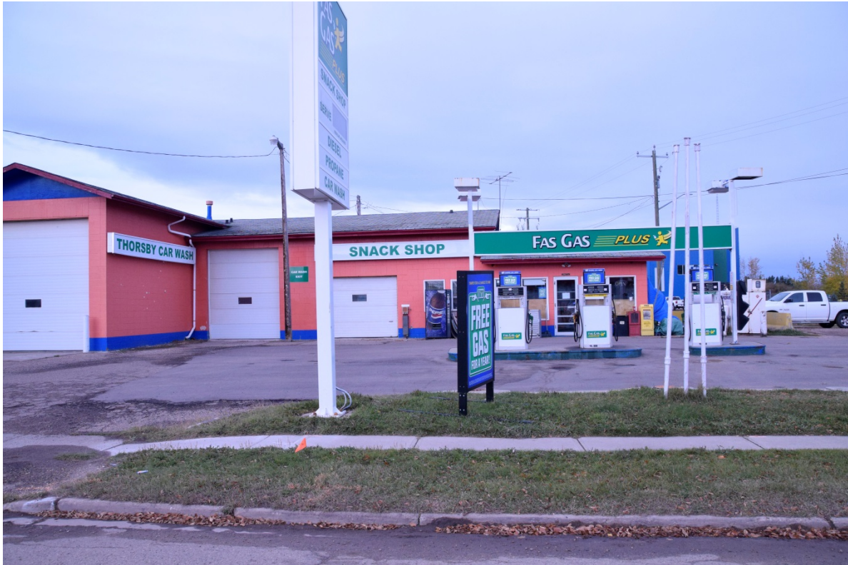
Figure 1: Thorsby Fas Gas Plus facing west
