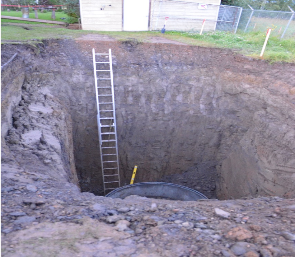
Figure 2. The ladder that the two labourers used to access the excavation.
