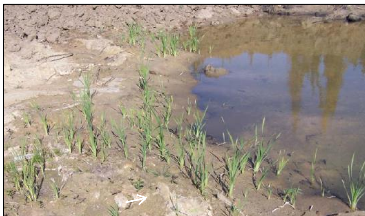
Figure 6.0 Constructed Wetland Features Young cattail shoots growing naturally; post construction
