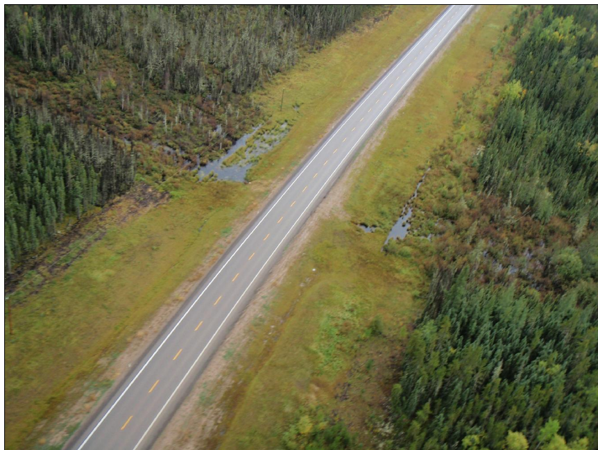
Photo 1 - Upstream aerial view of unnamed watercourse, at Highway 881 (September 2011).
