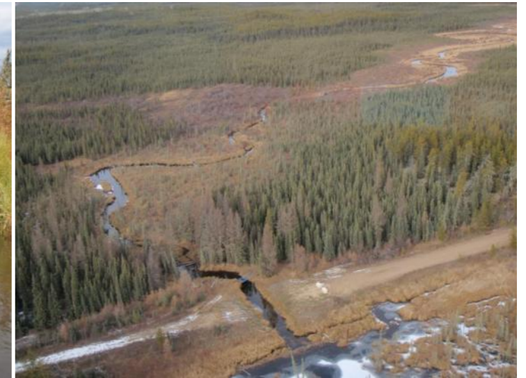
Photo 4: Downstream aerial view of crossing location, looking northeast (November 2011).
