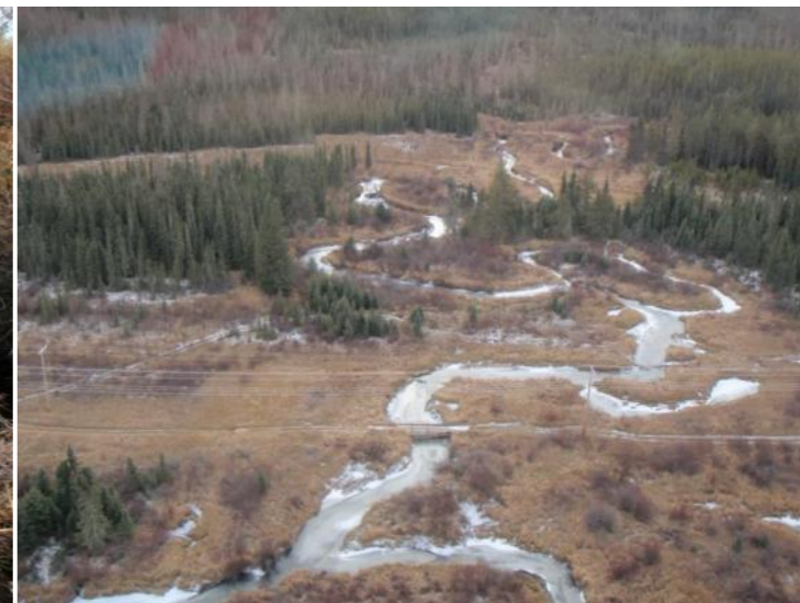
Photo 4: Upstream aerial view of crossing location, looking northeast (November 2011).
