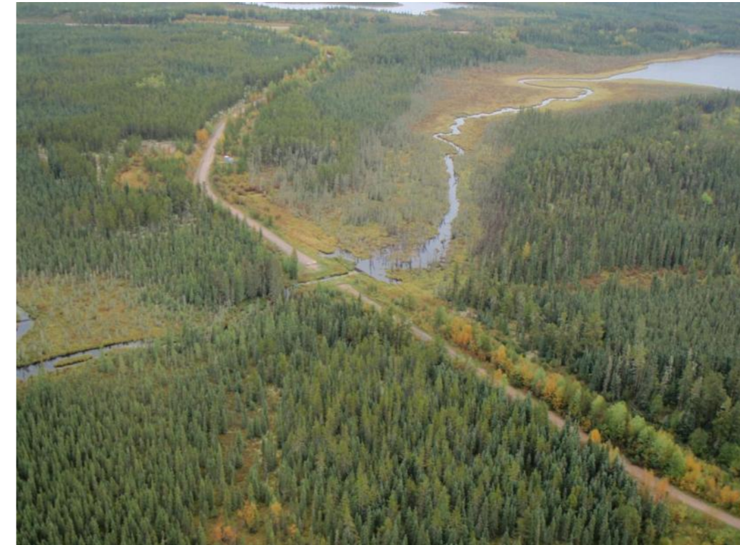
Photo 5: Aerial view of crossing location, looking upstream and northeast (September 2011).
