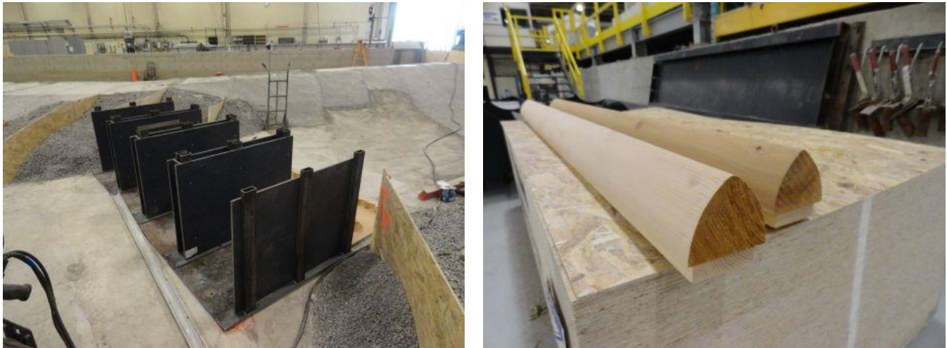
Figure 38. Left: diversion inlet pier struts and base plates installed in the basin. Right: precision milled hardwood pier noses after manufacture.
