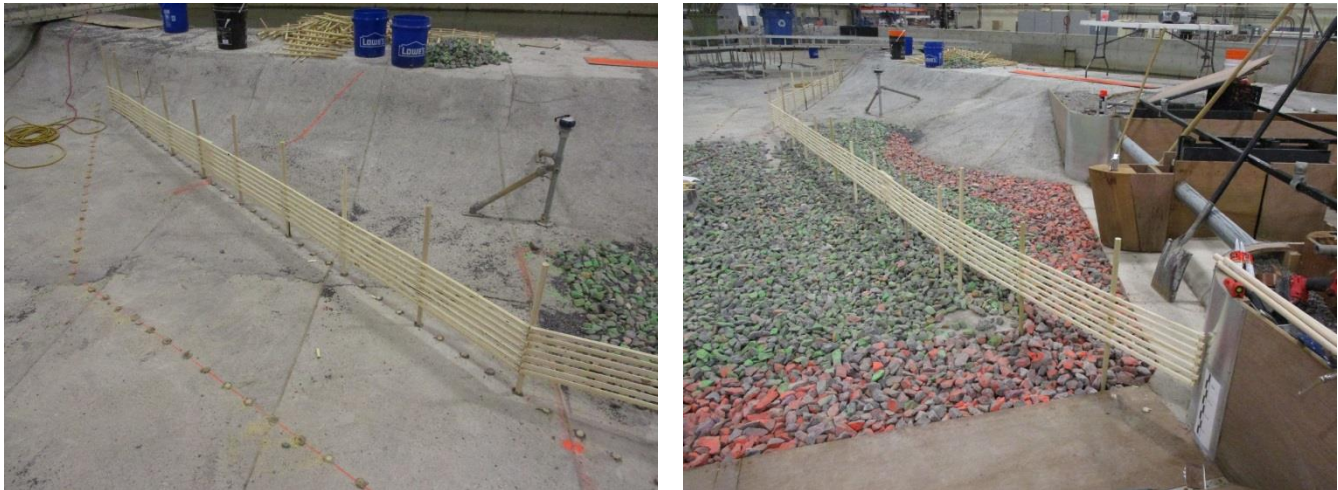
Figure 67. Debris Barrier F construction in the model.
