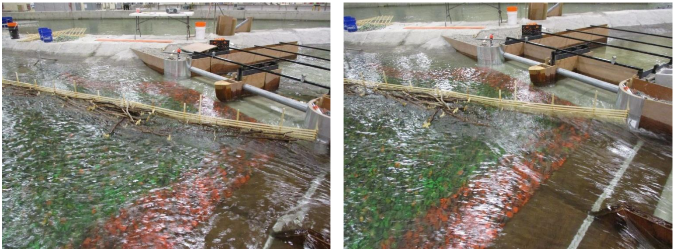
Figure 182. Gate operations to removed trees caught in debris barrier F. Left – dropping the LH Obermeyer gate to 1210 removed ~80 trees from the barrier. Right – lowering the diversion inlet gates and the RH Obermeyer gate removed ~15 trees from the barrier.
