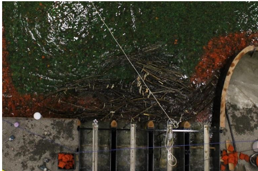
Figure 97. Debris jam of approximately 180 trees.
