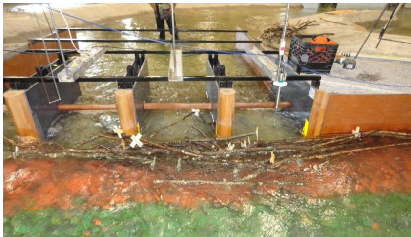
Figure 99. Collection of debris snagged on the diversion inlet piers.
