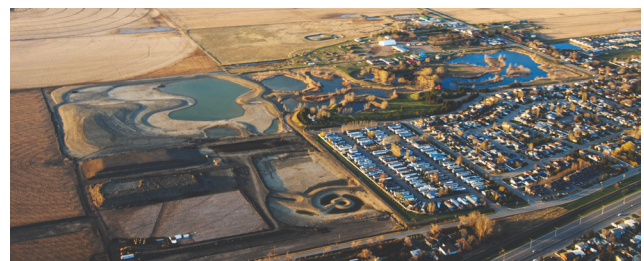
Northwest Constructed Wetland Complex, Town of Coaldale, Alberta.
