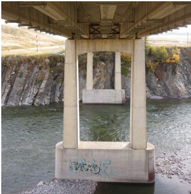
Figure 3: Concrete pier with shafts and arched cap.
