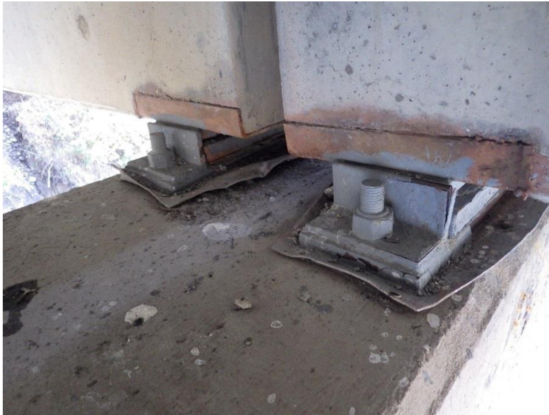
Figure 2: Steel sliding plate expansion bearings with self-lubricating bronze plates
