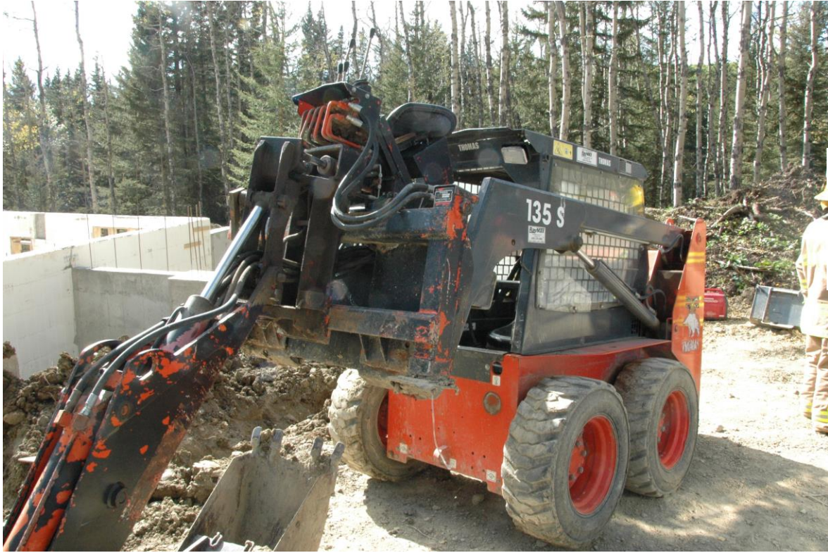
Photograph 2 – Shows the backhoe attachment and skid steer.
