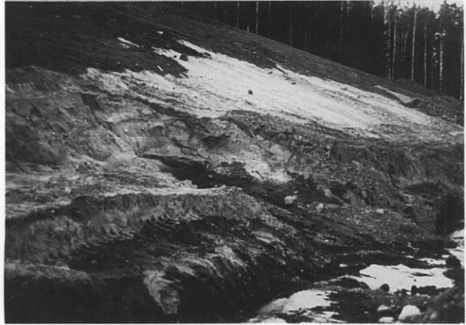
Plate 9. Bodies of sand and gravel incorporated within hummocky till. Groundwater discharge from these sand bodies causes problems for road construction due to slope instability (slump in foreground).
