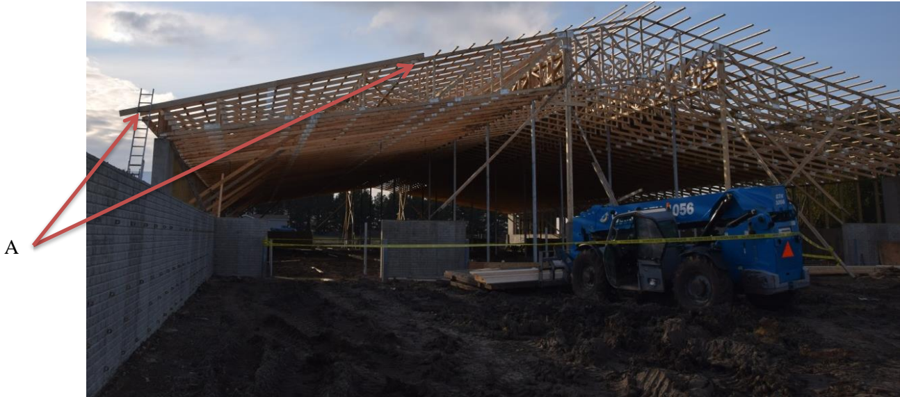
Figure 9. East end of dairy barn showing location of fascia board installation.
