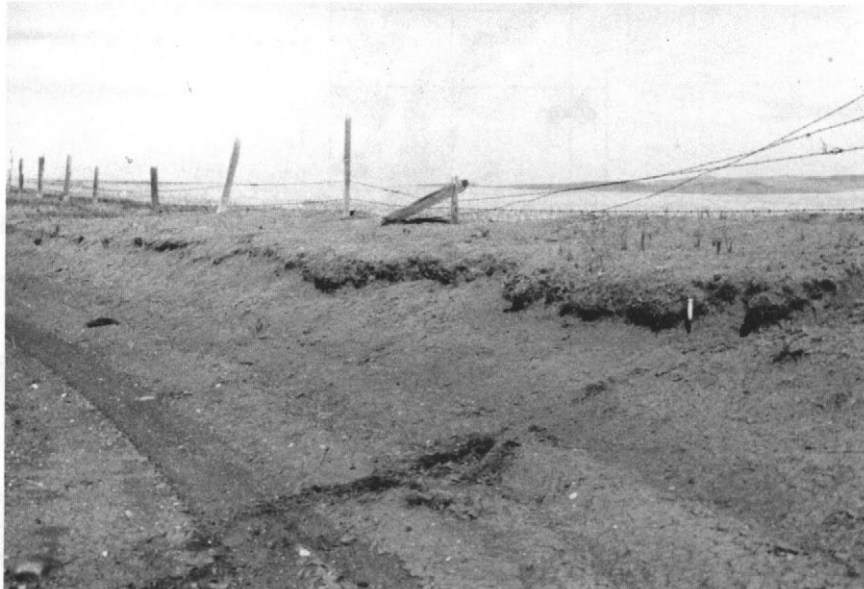
Figure 37. Evidence of wind eroded soils is often observed along fence rows.
