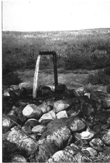
Fig. 3 —Artesian well. These wells (500 to 1,000 feet deep) are fed from an artesian basin that centers in this sheet.
