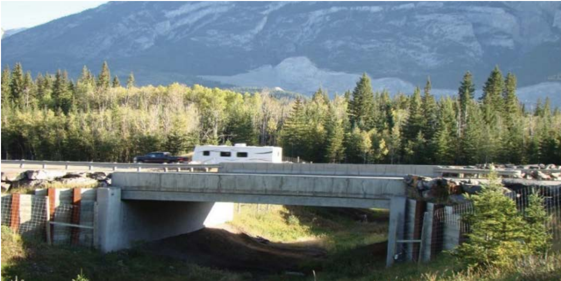
Figure 23. Trans-Canada Highway wildlife underpass near Dead Man's Flats, Alberta.
