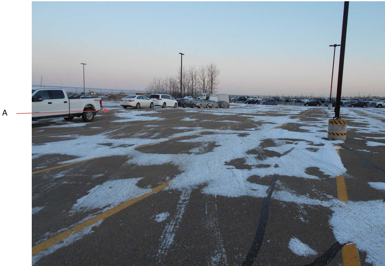
Figure 1. The parking lot and ground conditions at the time that OHS arrived on site, November 8, 2018.
