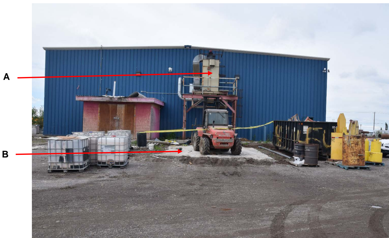
Figure 1. Work site at the back of the building
