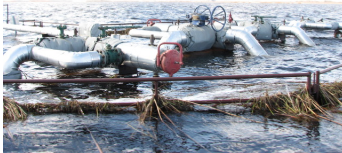
Figure 5-8. Consequences of planning activities using boundaries that were field delineated under dry and/or frozen conditions. Other considerations such as fluctuating wetland extents or lake levels, vegetative cover and soils were also not adequately investigated. Additional information and historical imagery was not appropriately identified or utilized to plan and avoid risks to infrastructure prior to undertaking the activity. Water levels were at a historic high when these photos were taken in 2011.
