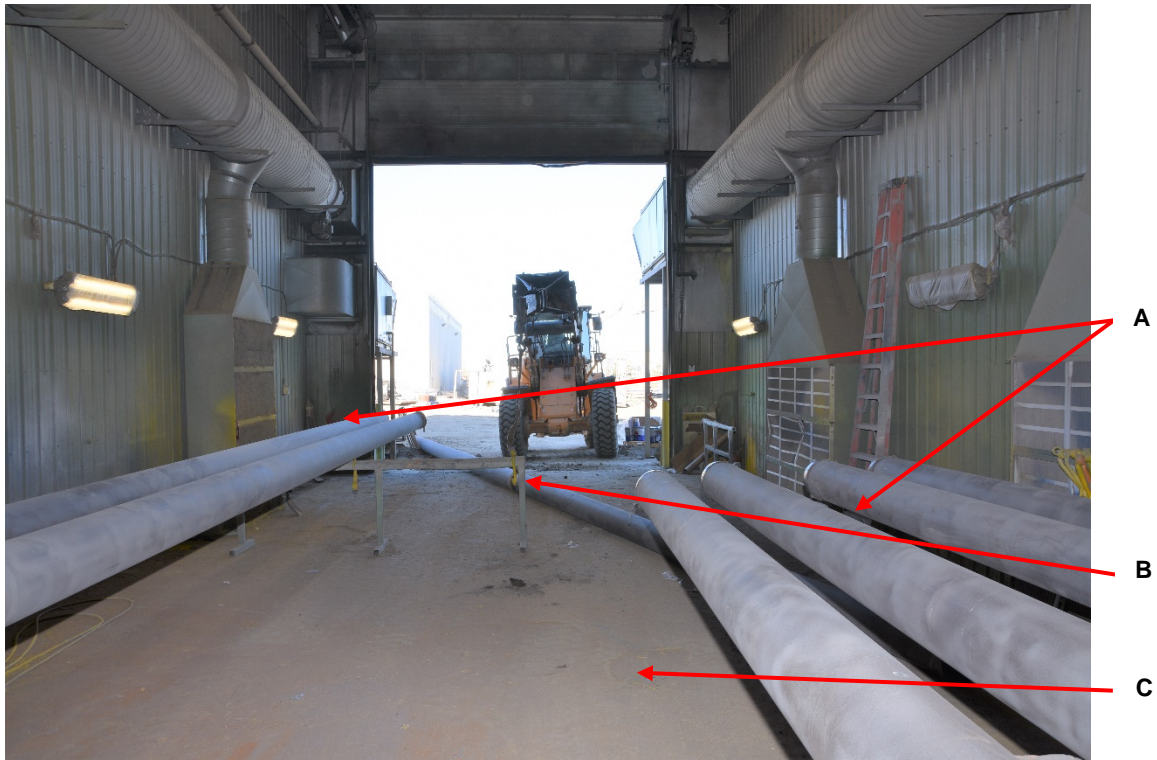
Figure 4. Interior of paint bay 4 with bunks and previously moved pipe sections.
