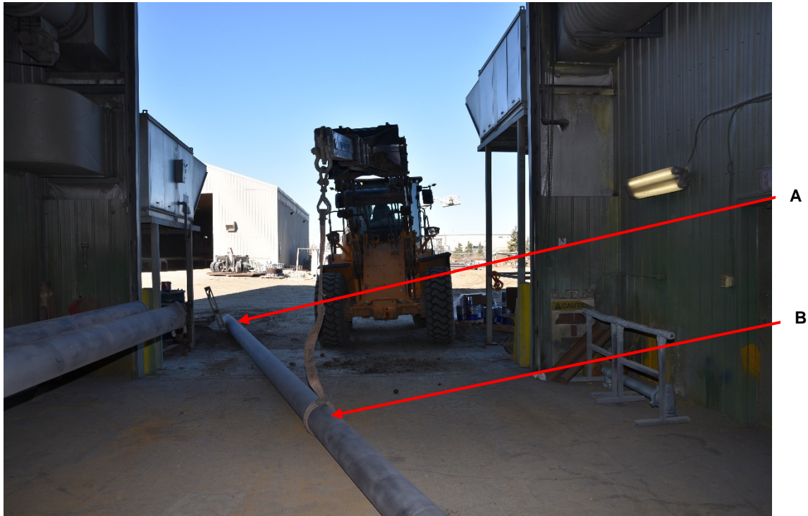
Figure 9. Section of pipe involved in incident.
