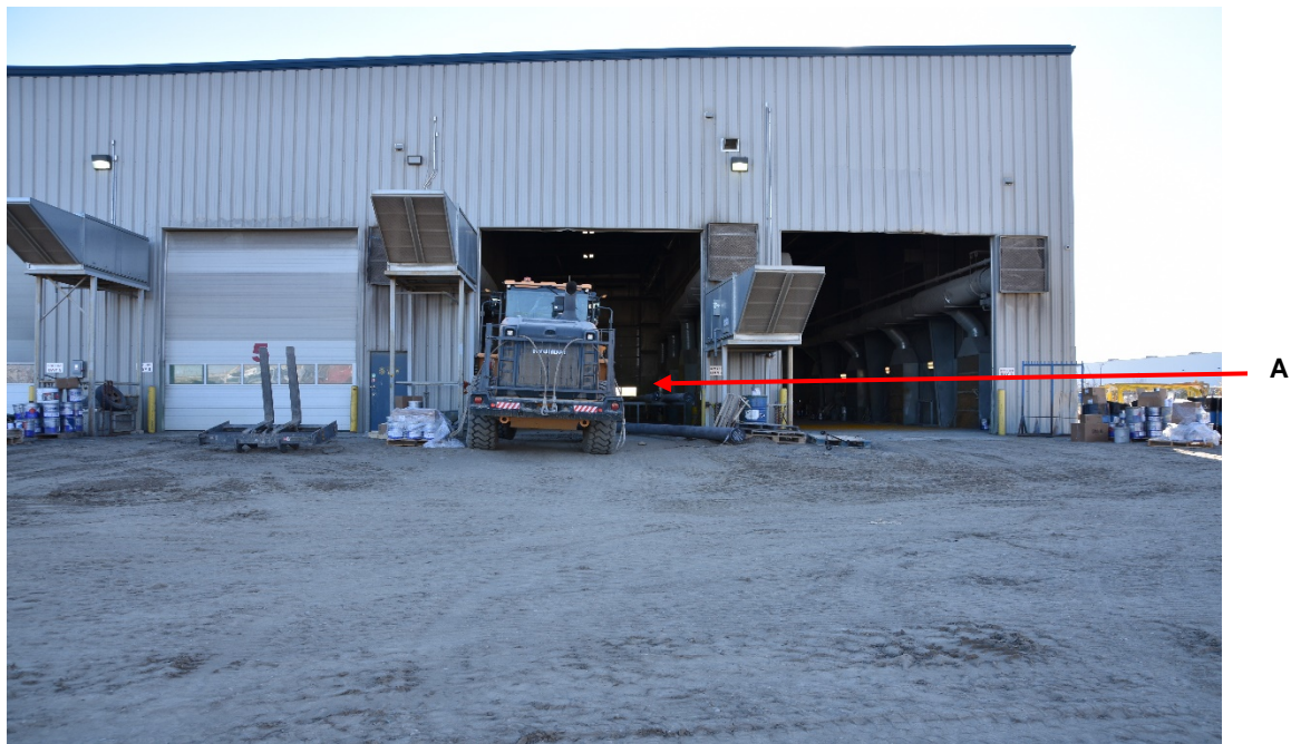
Figure 3. Paint bay 4 entrance.
