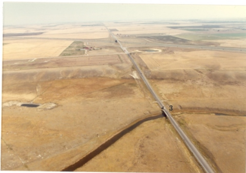
Site 3. Nose Creek At Calgary City Limits, On Secondary Highway #564, Aerial View Looking East
