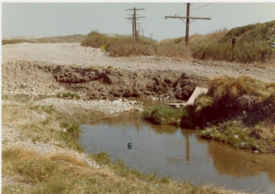
Site 6. West Nose Creek Above Confluence of Nose Creek, Ground View Looking North
