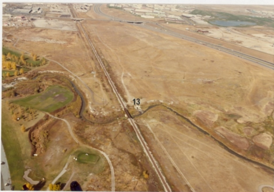
Storm Sewer N-13. Outfall Location on Nose Creek, Aerial View Looking North
