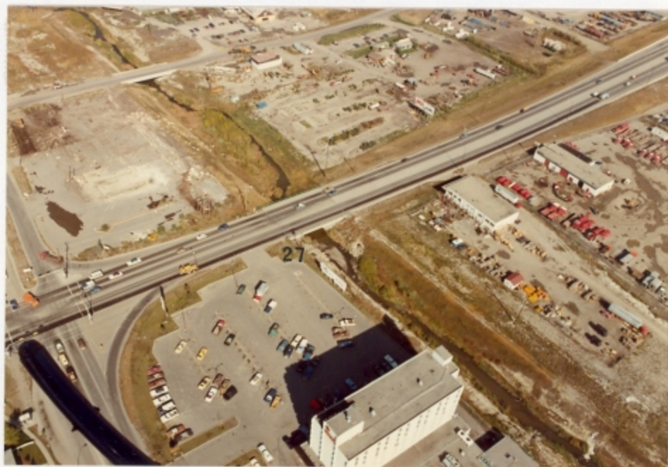
Storm Sewer N-27. Outfall Location on Nose Creek, Aerial View Looking Northeast
