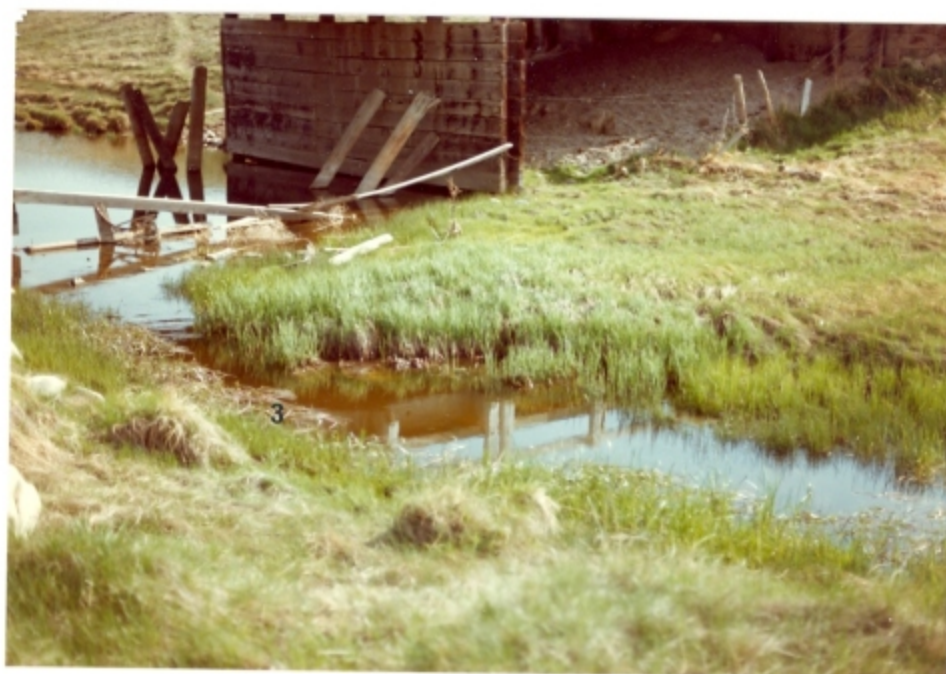
Site 3. Nose Creek At Calgary City Limits, Ground View
